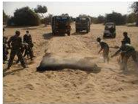
Construction of Expedient Road Bases
